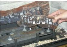
Place the Middle Left Log C)02-56 on the two pins as shown.
